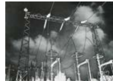
Fortunata Obrąpalska., Power Plant, photo: courtesy of the Asymetria Gallery
